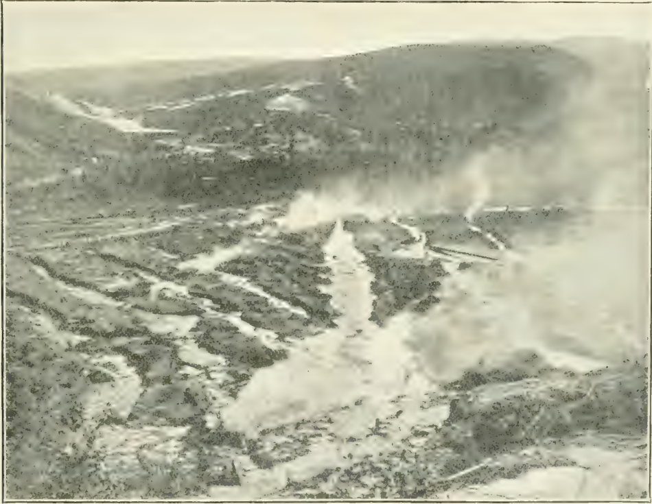
STRIPPING OPERATIONS ON CLAIM NO. 88 BELOW BONANZA. CREEK IN CENTRE AND CROSS-DITCHES IN 'MUCK.'
